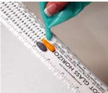
There are optimum mix consistencies that work best for any given application. The four most common consistencies I use are: slightly runny, slow moving, firm and extra dry.
